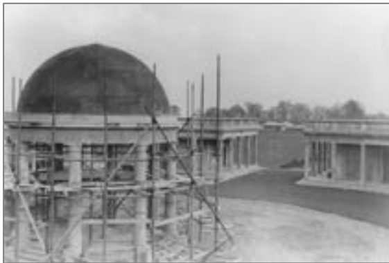
Construction of the bandstand dome
